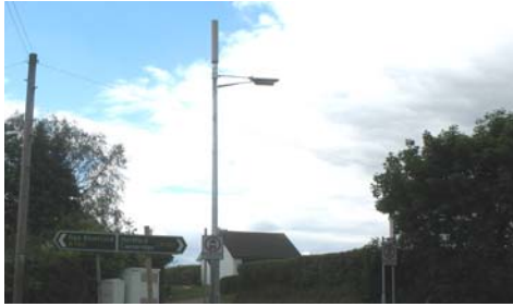
Photo 5: Example of replacement street light incorporating a base station (Source: Agent, T-mobile)
