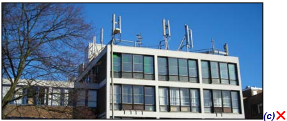
Photo 3: Camouflage - (a) and (b) Antennas disguised to blend in with building features (source: Stappard Howes, Chertsey, Surrey) (c) Overly prominent or multiple antennas detract from streetscene (Summertown, Oxford)
