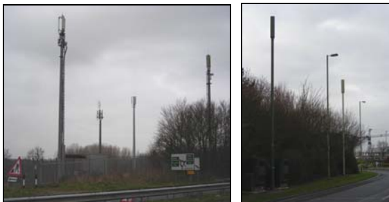
Photo 6 (a) & (b): Multiple masts can cause unacceptable clutter (examples in Oxford area)
